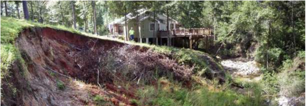
Recent mass wasting of streambank in Lake Forest. Site DA23a.
