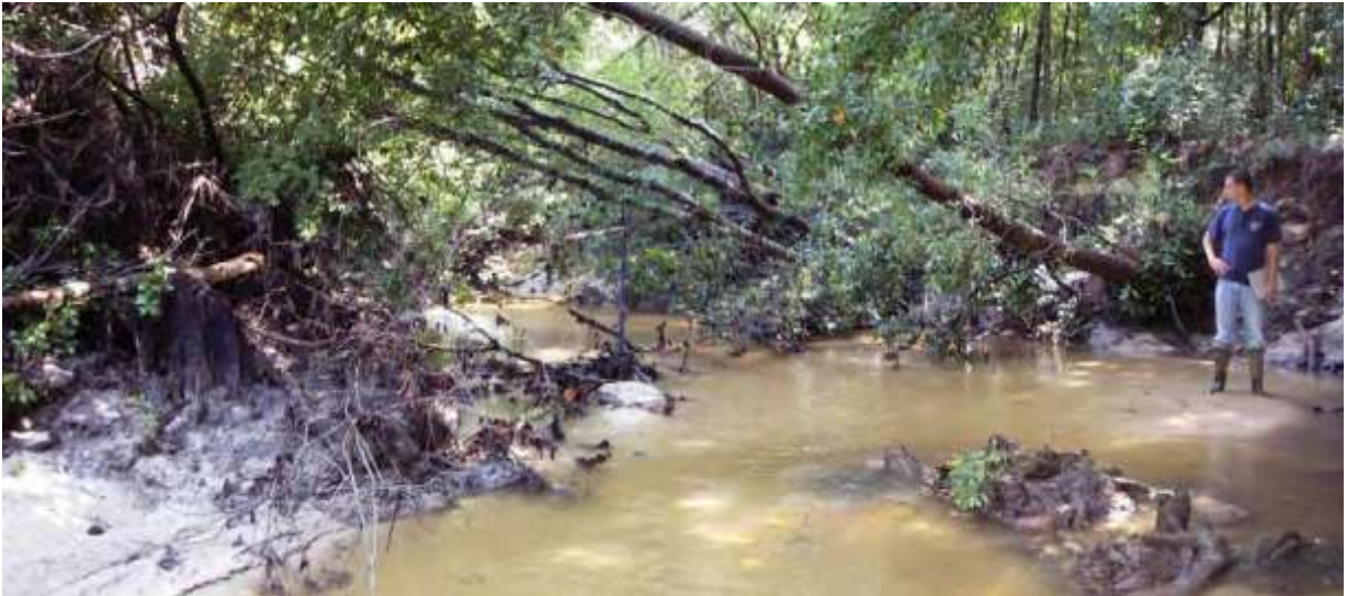
Trees recruited to channel by bank mass wasting. Site D5.
